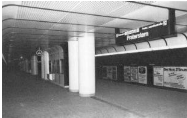
Subway station in Vienna; note the perforated metal facing for the sound absorptive ceiling treatment.
