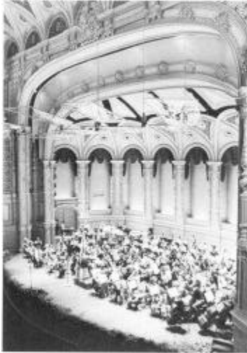
Figure 1. As an example of the first application, the curved surfaces above the stage of the Orpheum Theatre, Vancouver, B.C., are made of finely perforated metal sheet, not of plaster as they appear. The perforations allow the sound to pass through and to reflect back into the hall at desired locations, from specially designed surfaces behind the perforated metal.
