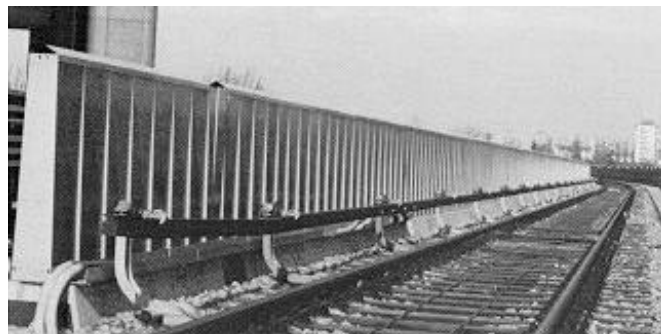
Figure 28. Sound absorptive treatments in the station. A. Indicates the absorptive surfaces -- j to m, as shown; n, 35 meters of sound absorptive walls in the tunnel. B. Reverberation time in the station. C. Effective sound level of the passing trains.
