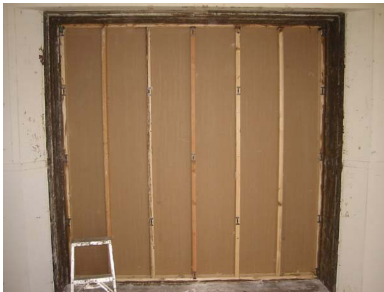
Figure 2: Green Glue® Noiseproofing Clip RC Layout Photo
